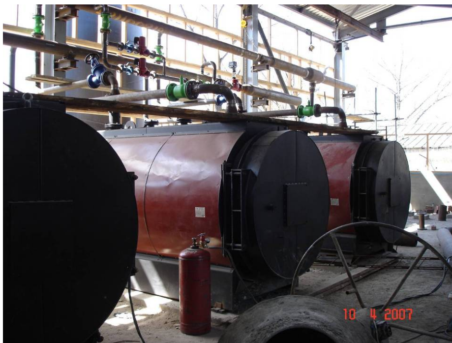
Fig. A.4-8. Assembling of three ZIOSAB-2000 peak-load hot-water boilers at HPS-1
