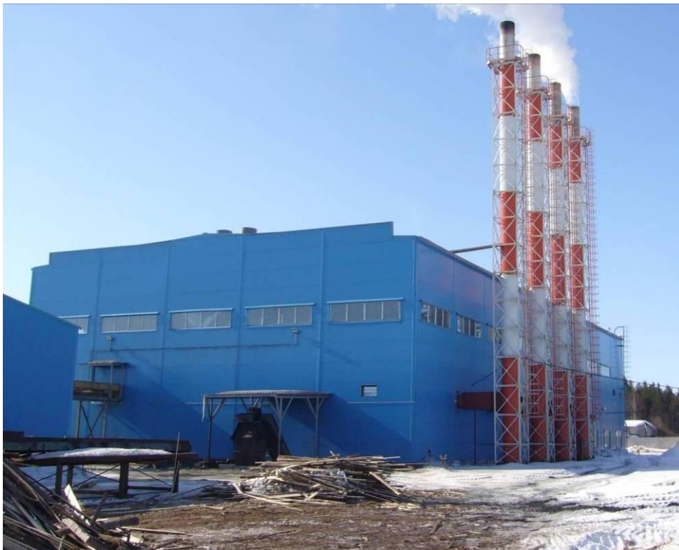
Fig. A.4-5. New biofuel boiler house
