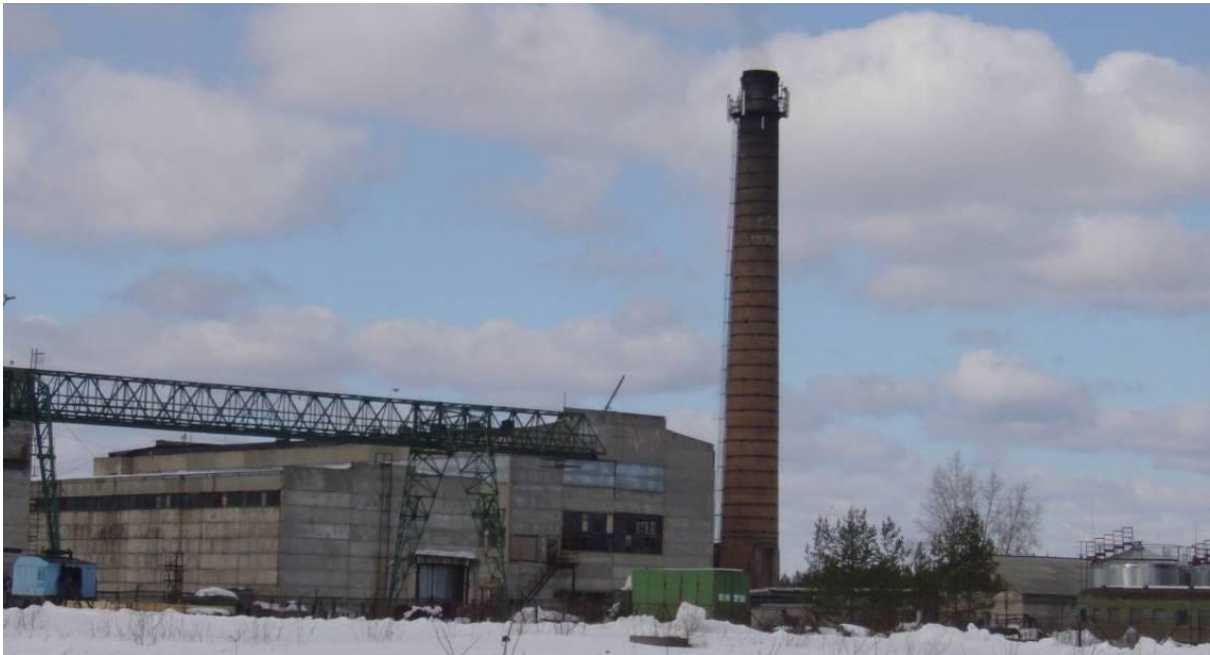
Fig. A.4-3. Residual fuel oil boiler house owned by OJSC “SBM”
