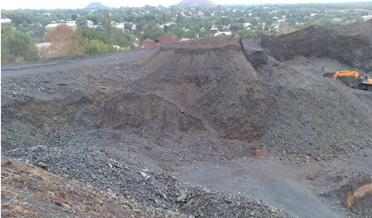
Figure 2 - The exterior of the waste heap under dismantling stage
