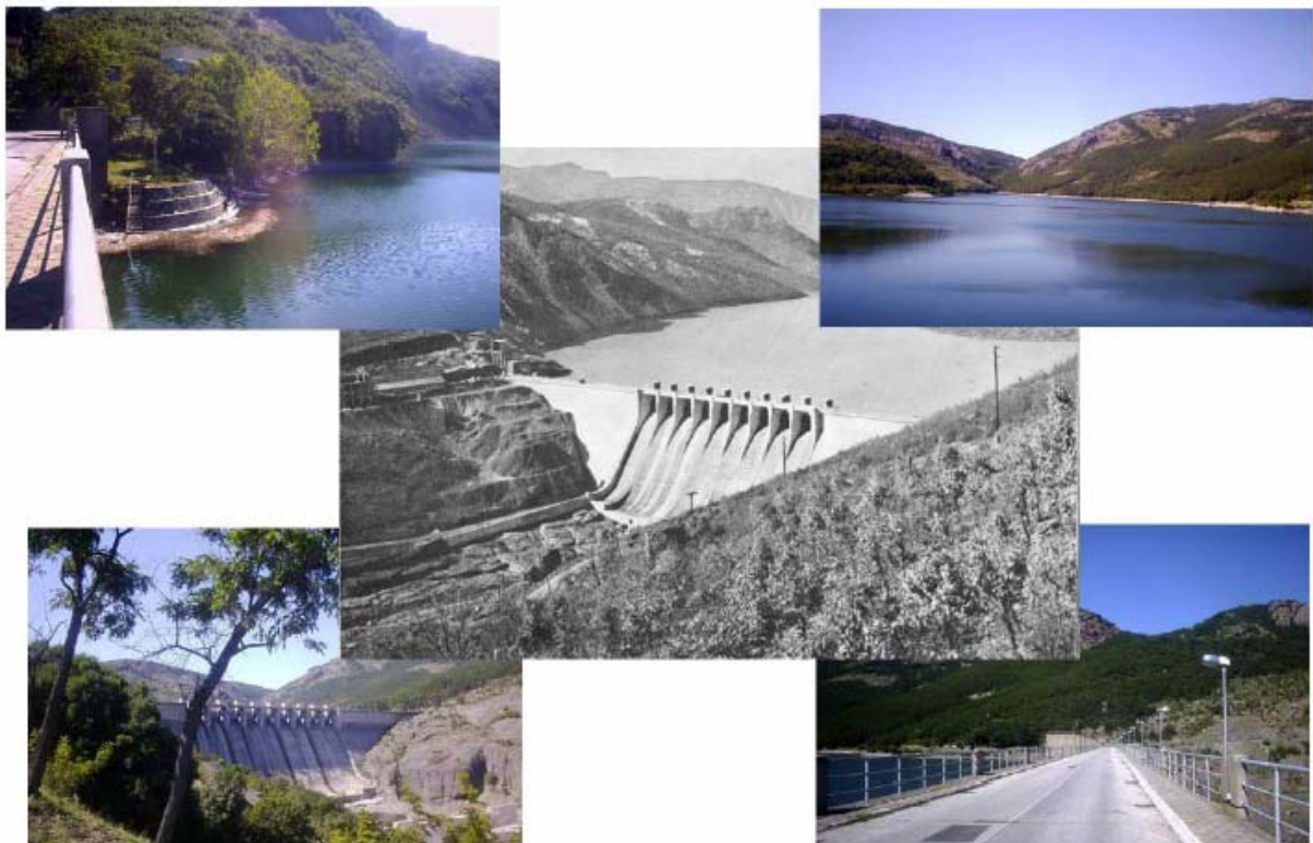
View of Studen Kaldenets Reservoir
