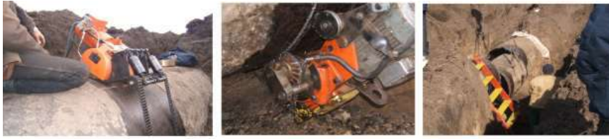
Figure 3. Cutting off the damaged pipeline section
