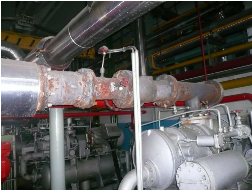
Picture 2.7. Ammonia refrigeration compressor
