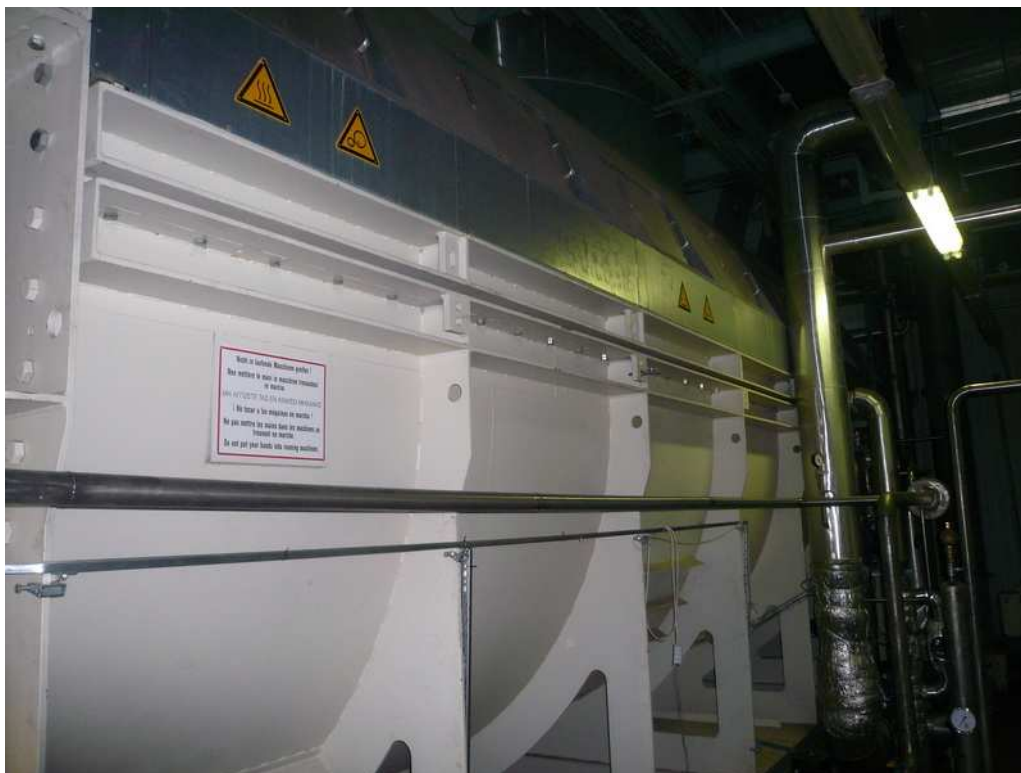
Picture 2.13. The building of drier of beer wort
