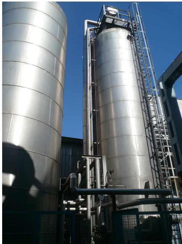
Picture 2.3. Capacity to collect carbon dioxide that comes from fermenting tanks
