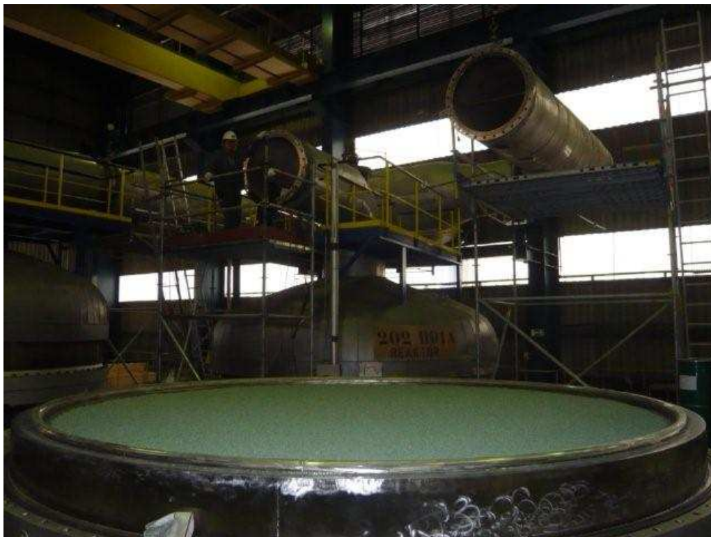
Figure 2: Installation of secondary catalyst
