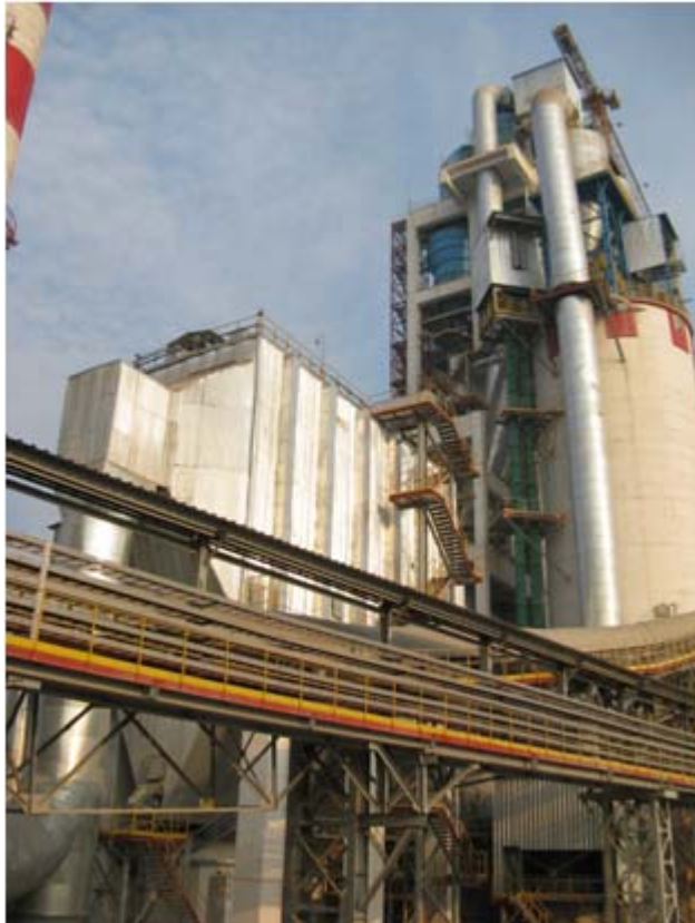
Figure 6: New cyclone pre-calciner
