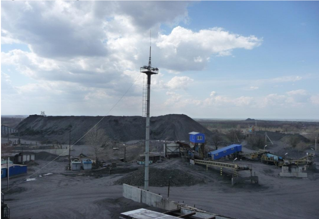
Figure 4. Waste heap of the former mine #40.
