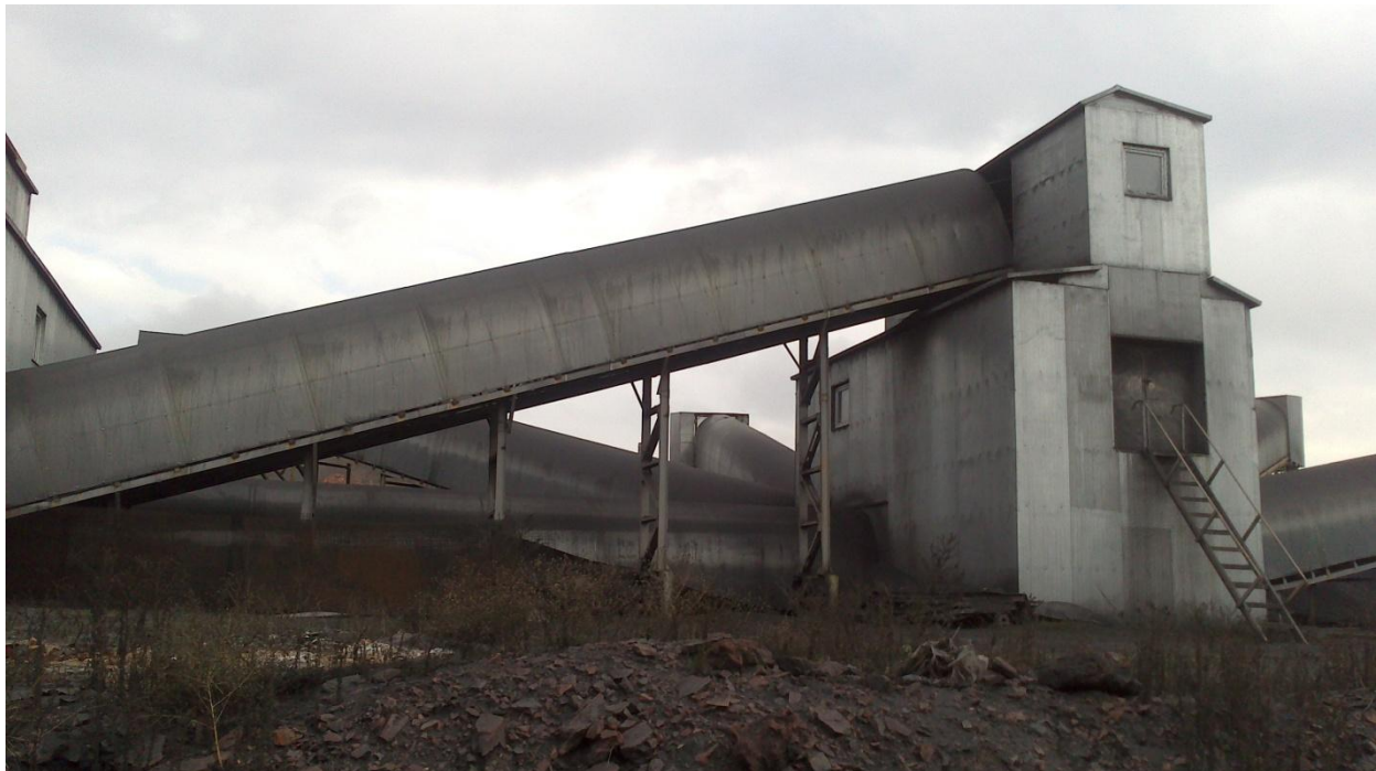
Figure 3 - Equipment for the rock mass sorting
