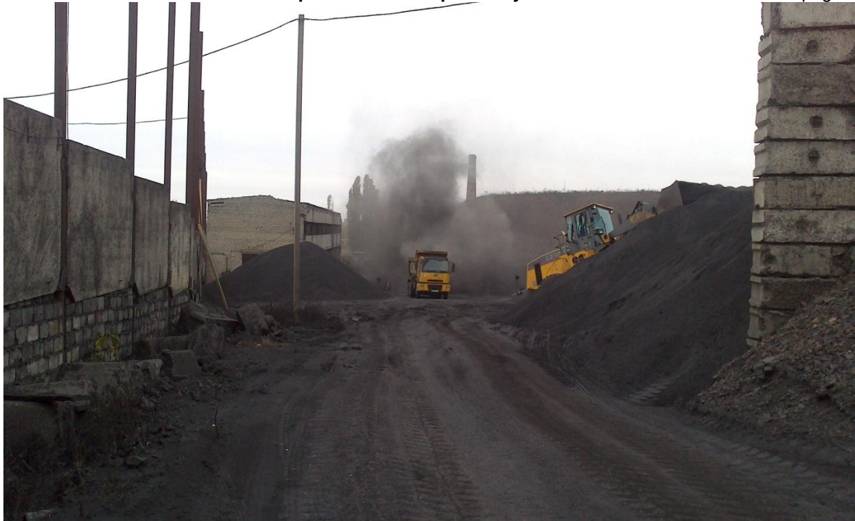
Figure 4 - Machinery involved in the project.
