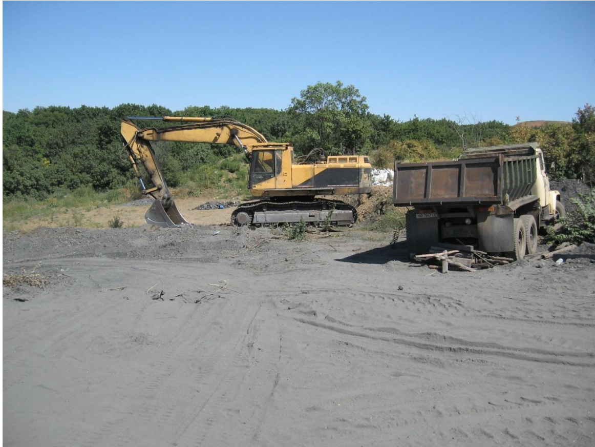
Figure 4 - Machinery involved in the project.
