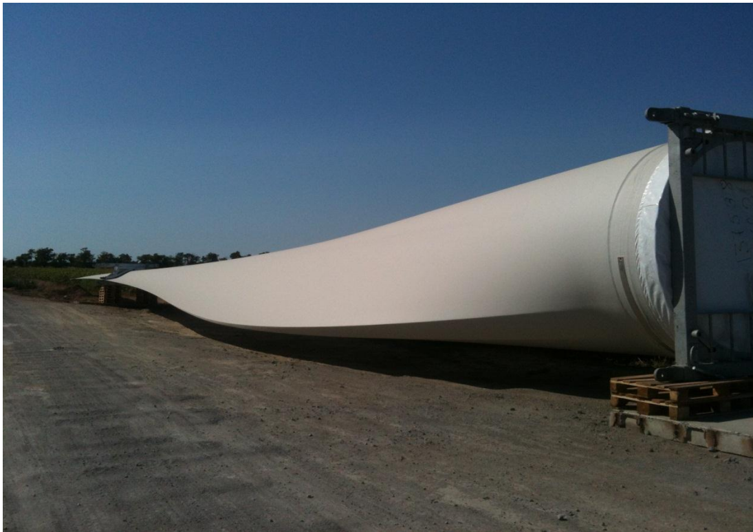
Figure 5. Vestas V112-3.0 turbines blade on the project site
