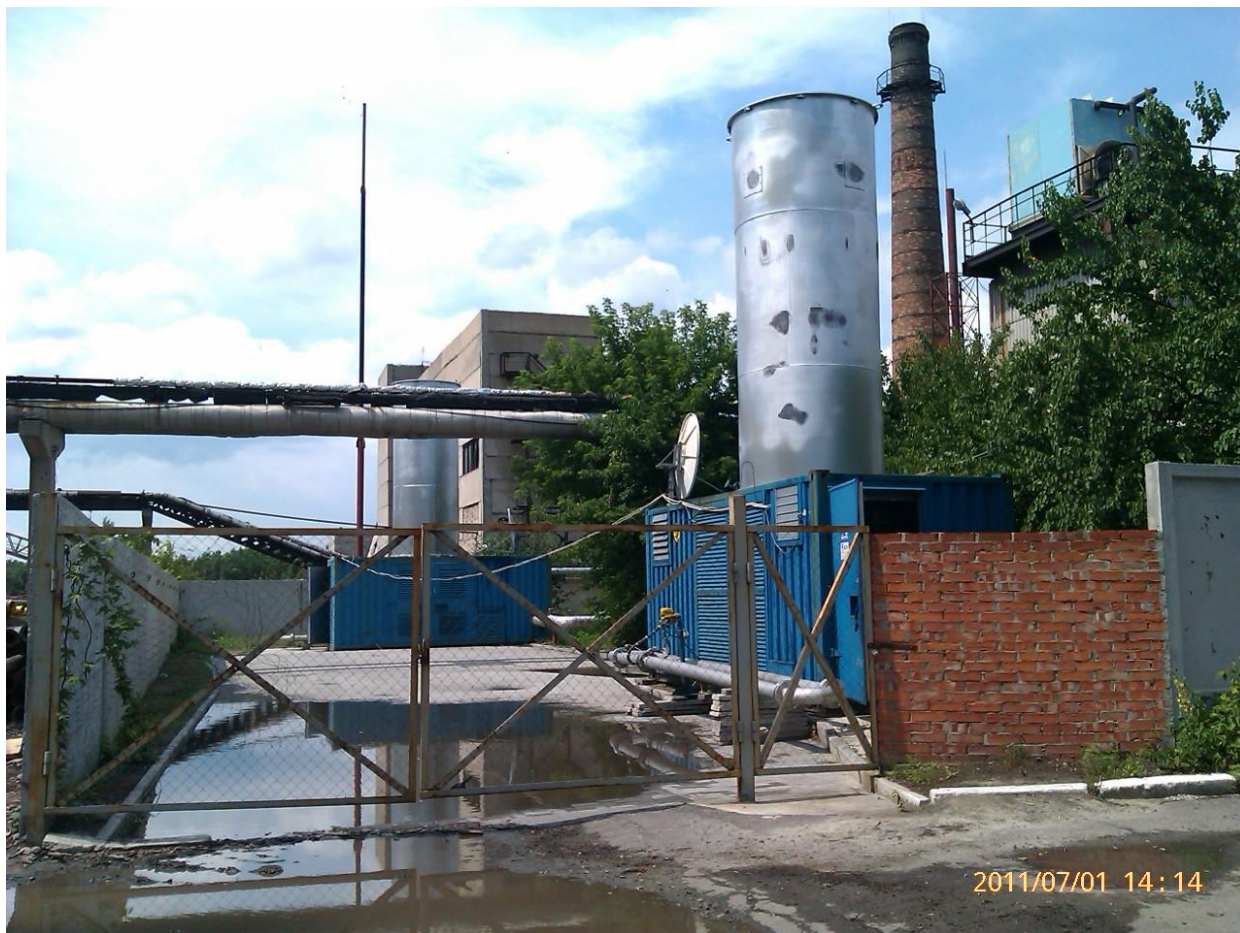
Figure-4 Flare 3 and Flare 4 – DTEK MINE KOMSOMOLETS DONBASSA PJSC, Air Shaft Nr.3
