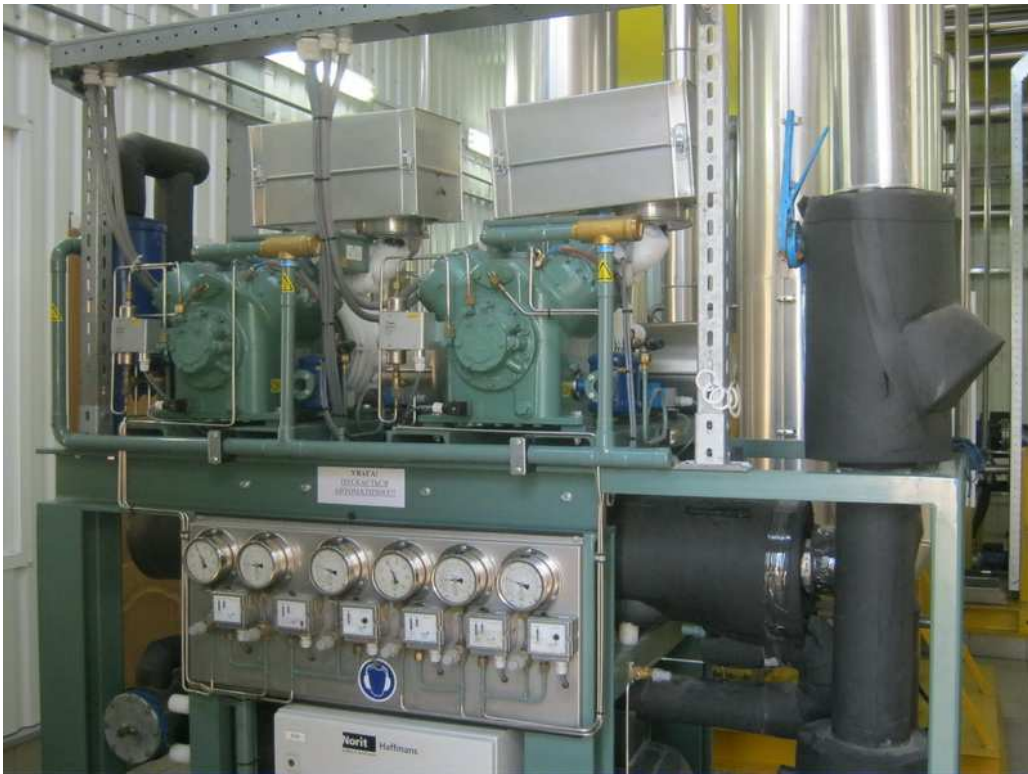
Figure 9 Equipment for preparation of liquid carbon dioxide “Haffmans B.V.”, Netherlands
