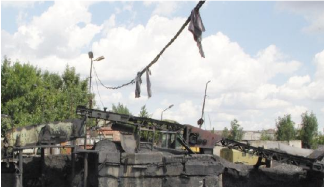
Figure 4 - Machinery for sorting the rock mass
