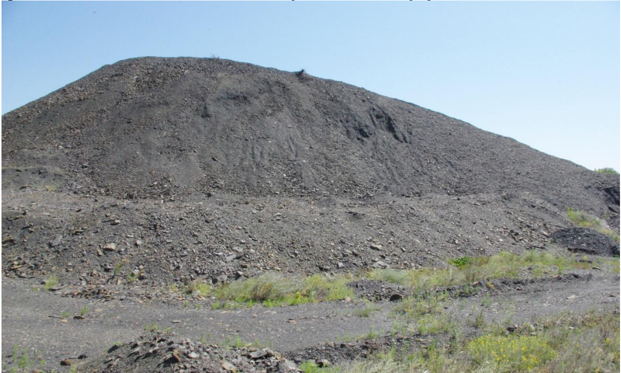
Figure 2 - The exterior of the waste heap of “Novopavlovská” mine under dismantling stage
