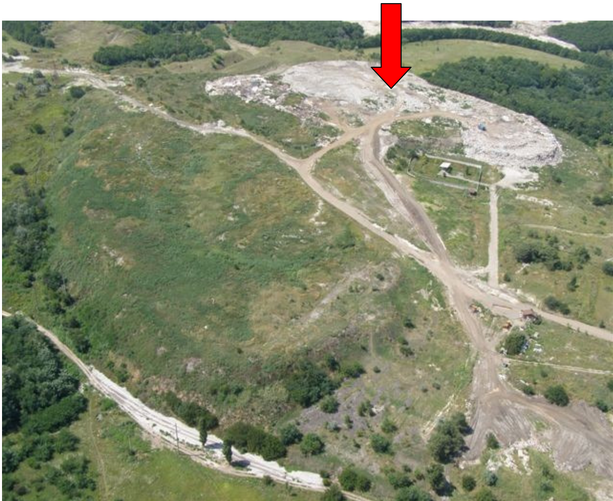
Figure 3 shows an aerial shot of the site
