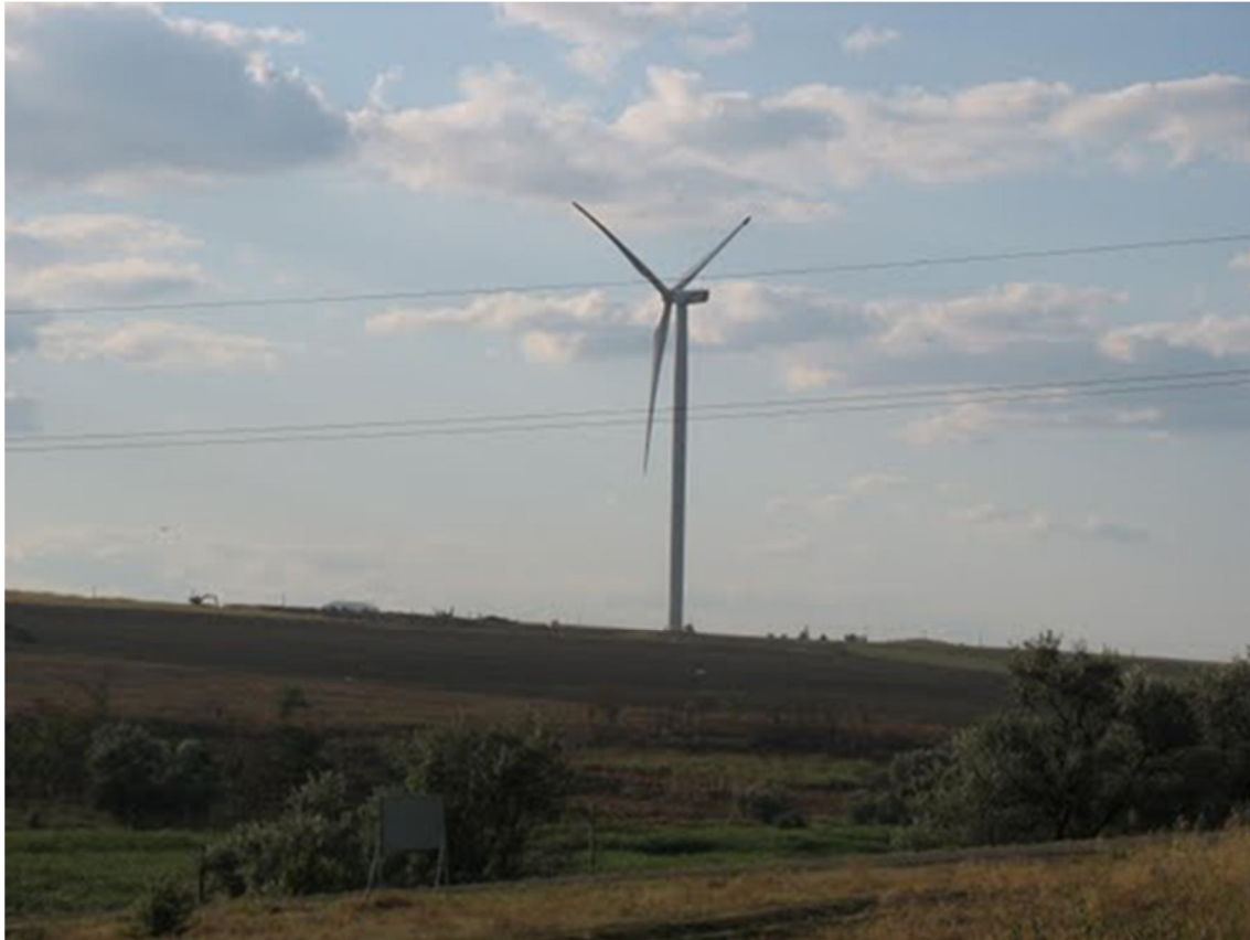
Figure 3. Wind power turbine FL 2500 installed at project site
