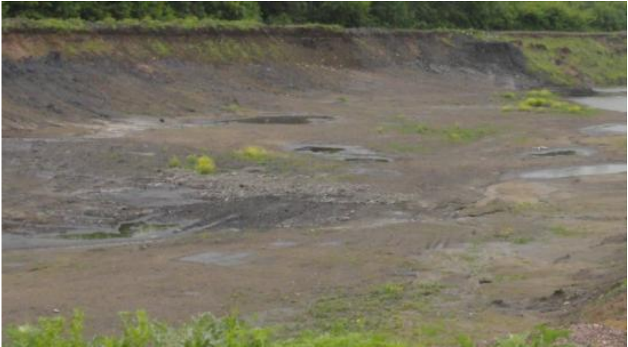
Figure 2 - Slurry pond involved in the project
