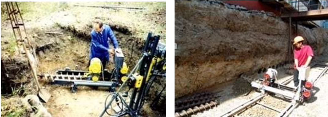
Figure 4. Operation of horizontal drilling machine
