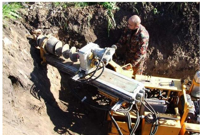
*Figure 4. Operation of horizontal drilling machine*
