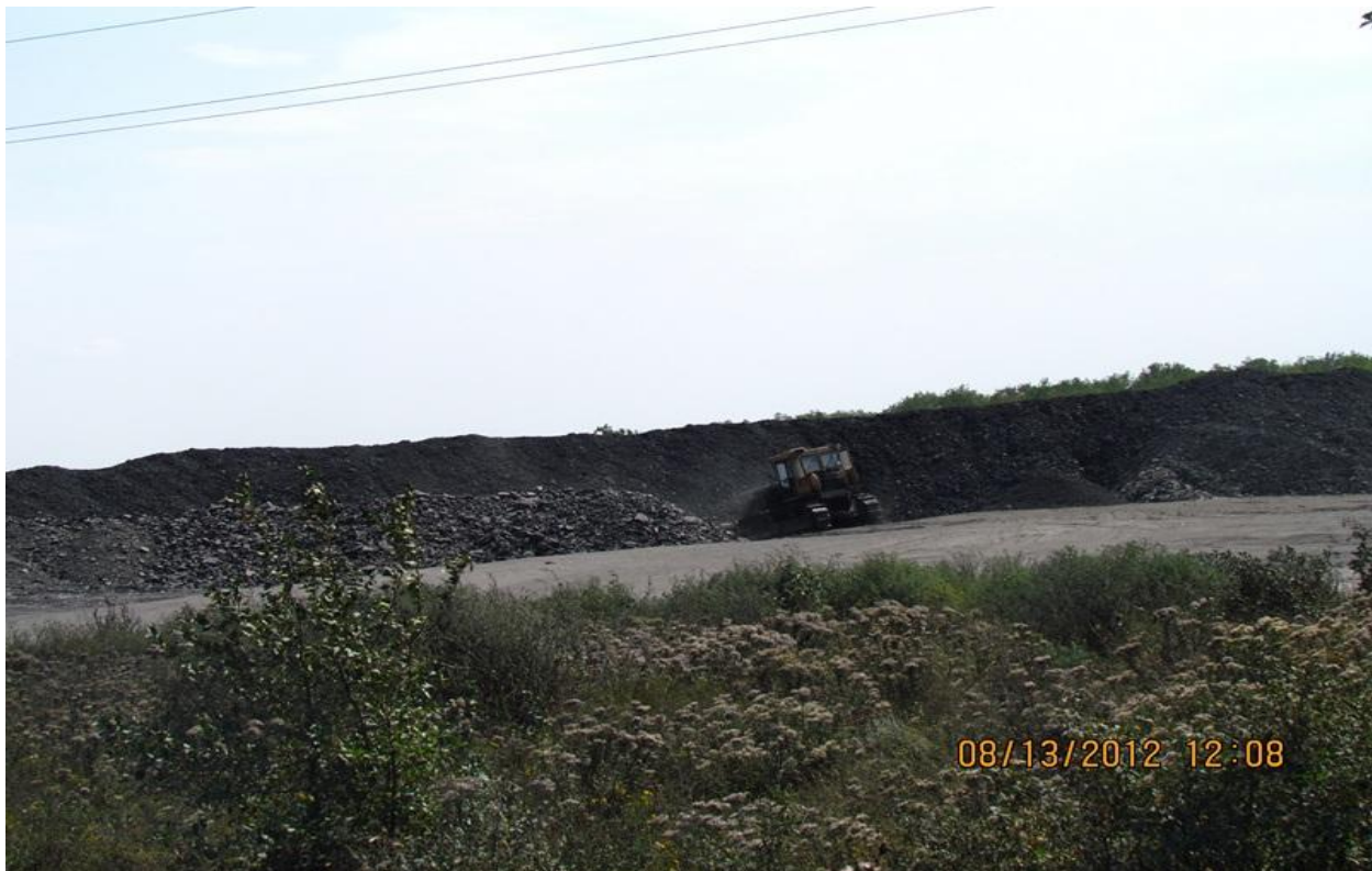
Figure 3 - The exterior of the waste heap#1 at mine #3 under dismantling stage
