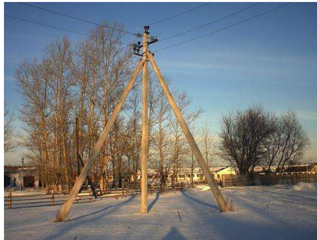
Figure 8. Towers of overhead power lines
