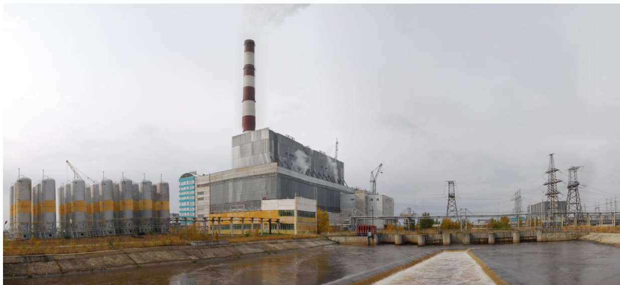
Figure A.4.1.2 – Photo of Nizhnevartovsk State Regional Power Plant
