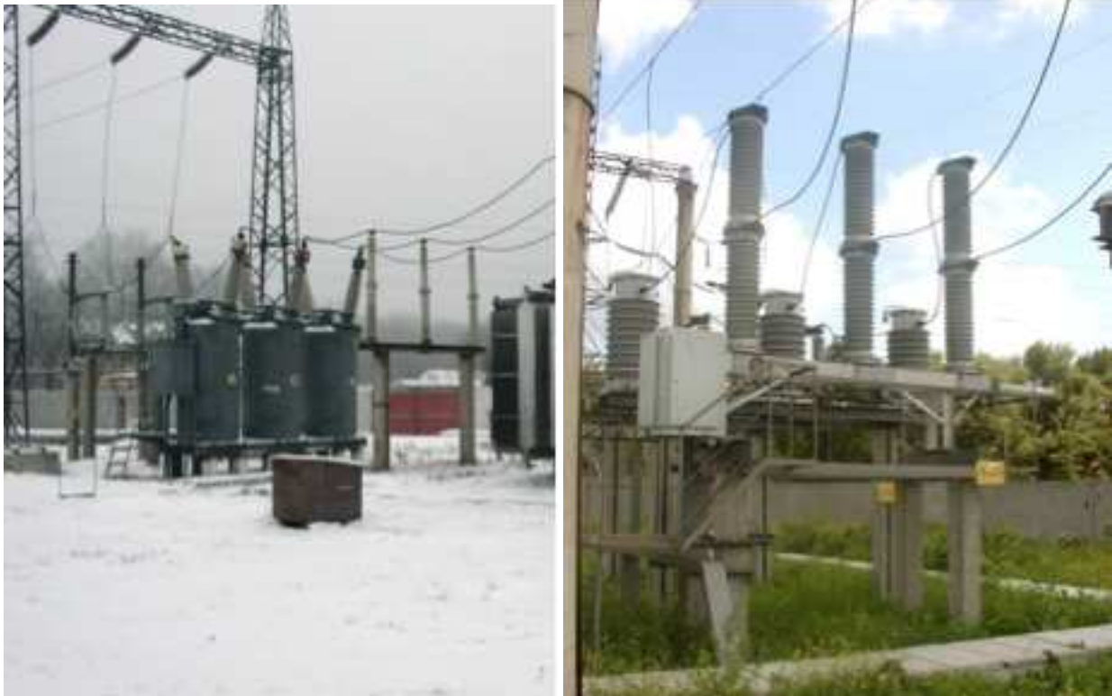
Figure 8. The Circuit Breakers before and after the Reconstruction.
