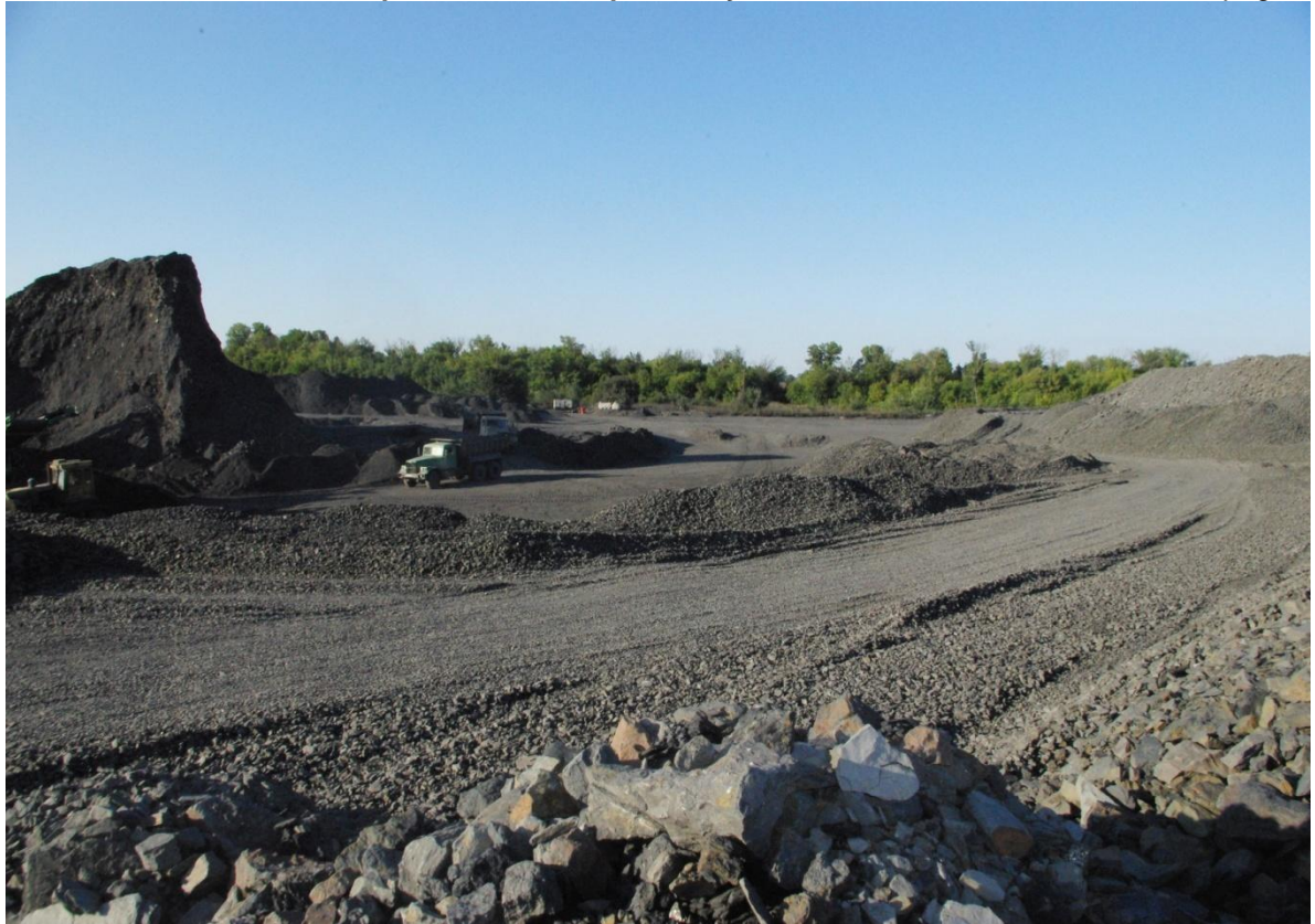
Figure 3 - The exterior of waste heap under dismantling stage
