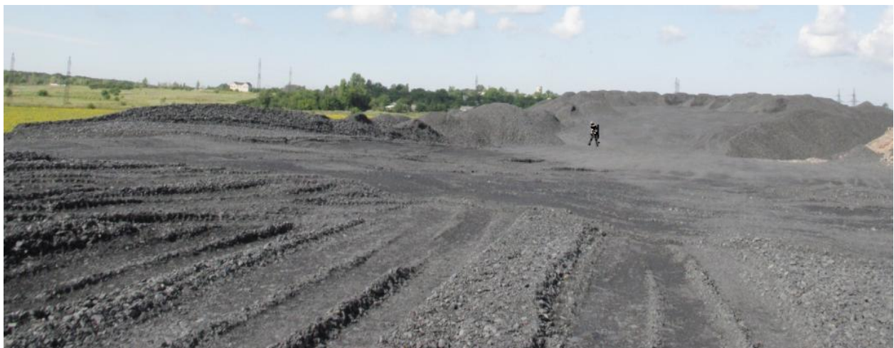
Figure 3 – The waste heap under final stage of dismantling.
