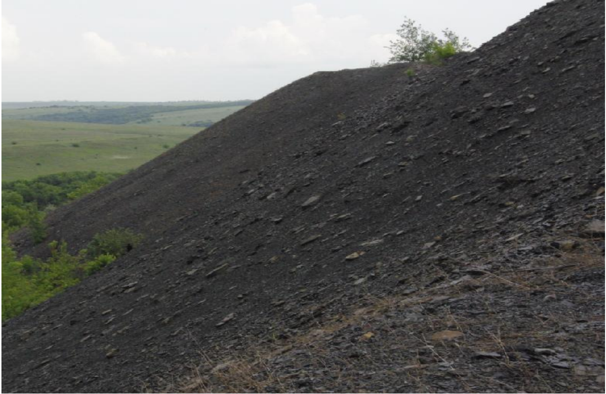
Figure 2 - The exterior of the waste heap under stage of dismantling
