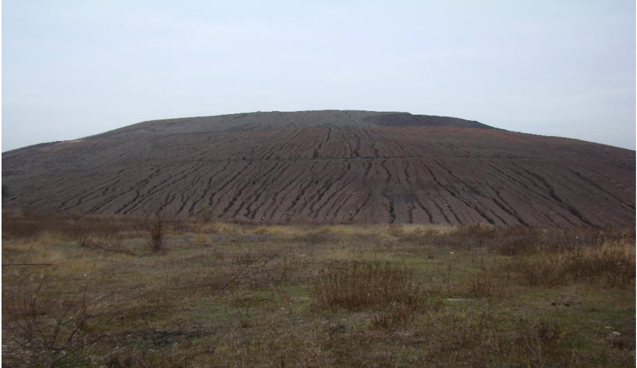
Figure 2 – Waste heap under dismantling stage
