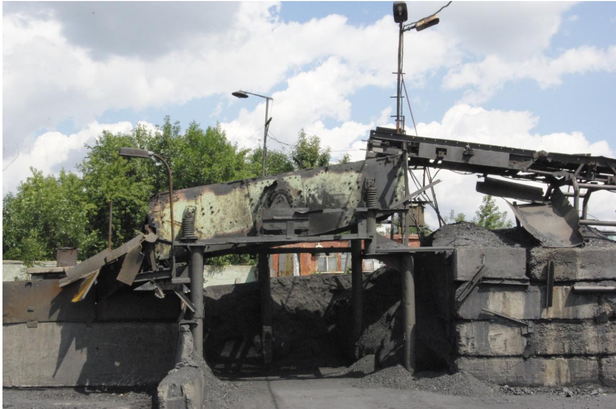
Figure 4 - Machinery for sorting the rock mass
