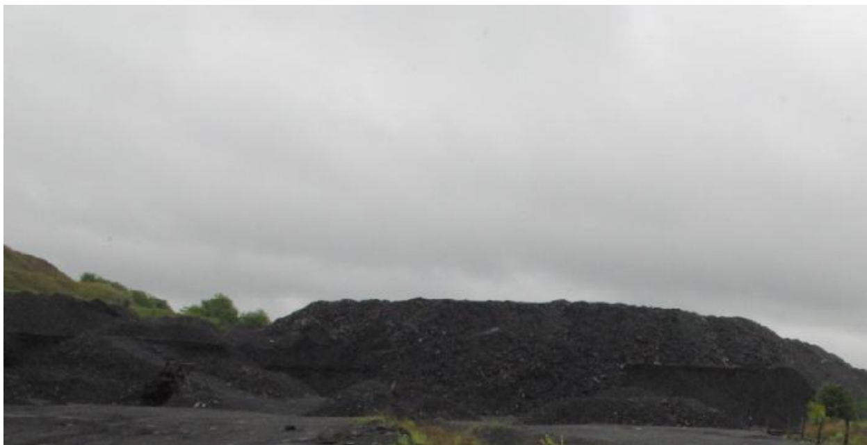
Figure 3 – Exterior appearance of the waste heap under dismantling stage
