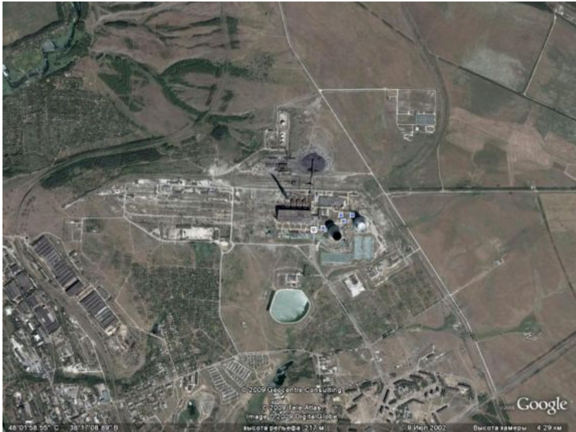
Figure 3: Power plant satellite view 10 .
