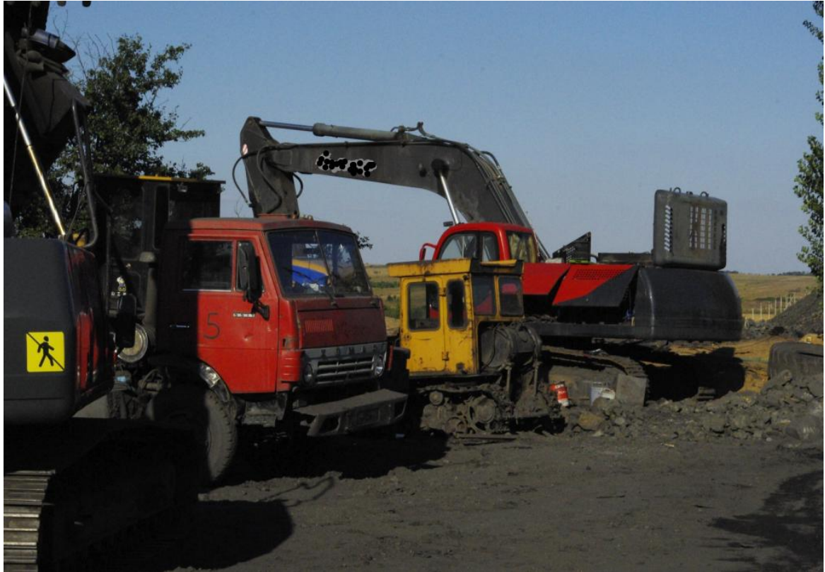
Figure 5 - Machinery involved in the project and weight scales.
