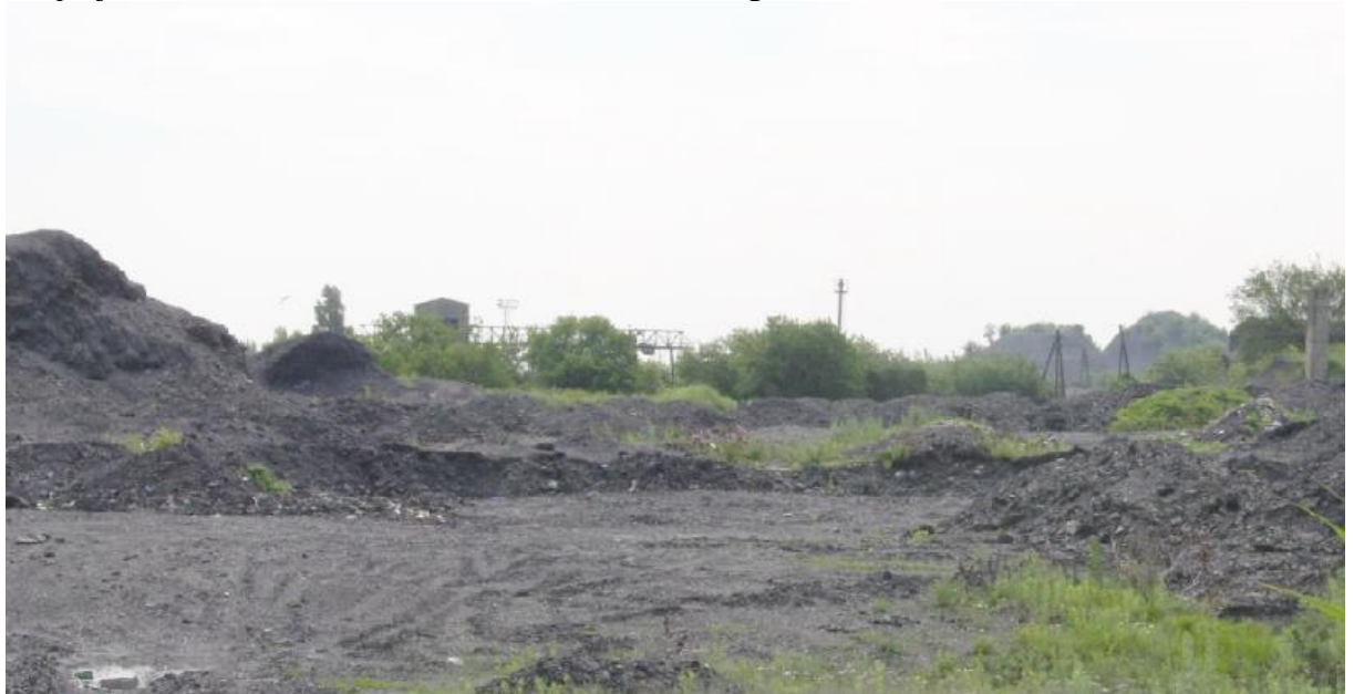
Figure 2 - The exterior of the waste heap under stage of dismantling
