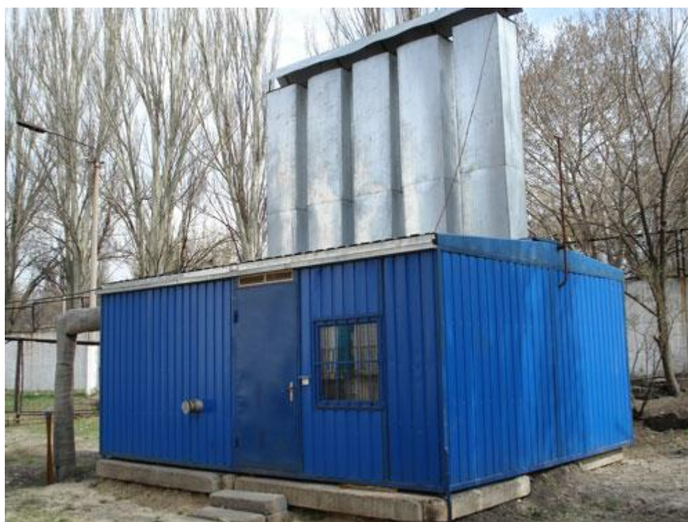
Figure. 3. Boiler Mini-Don of 94% coefficient of efficiency
