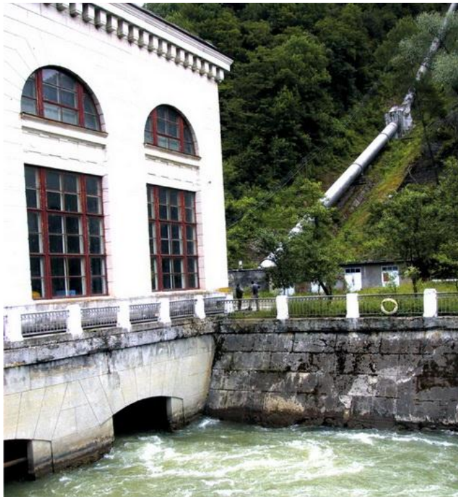
Figure 3 – Main building of Tereblya-Ritska HPP and pressure piping.
