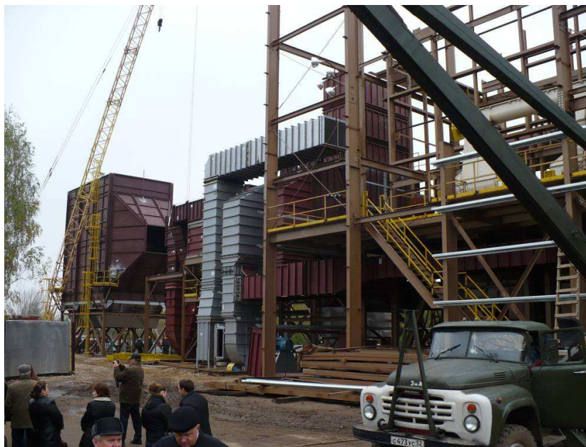
Fig. A.4-2. Erection of the boiler house equipment
