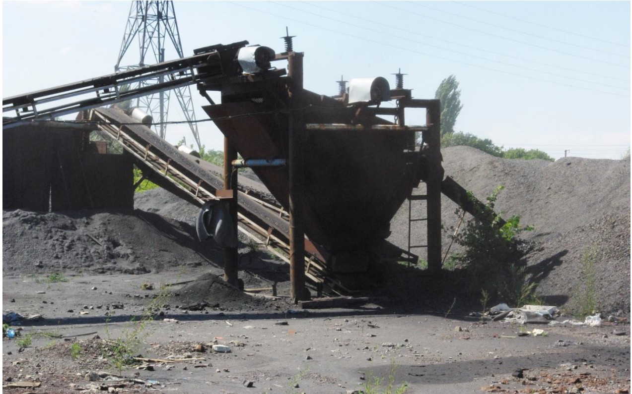
Figure 4 - Machinery for the rock mass sorting
