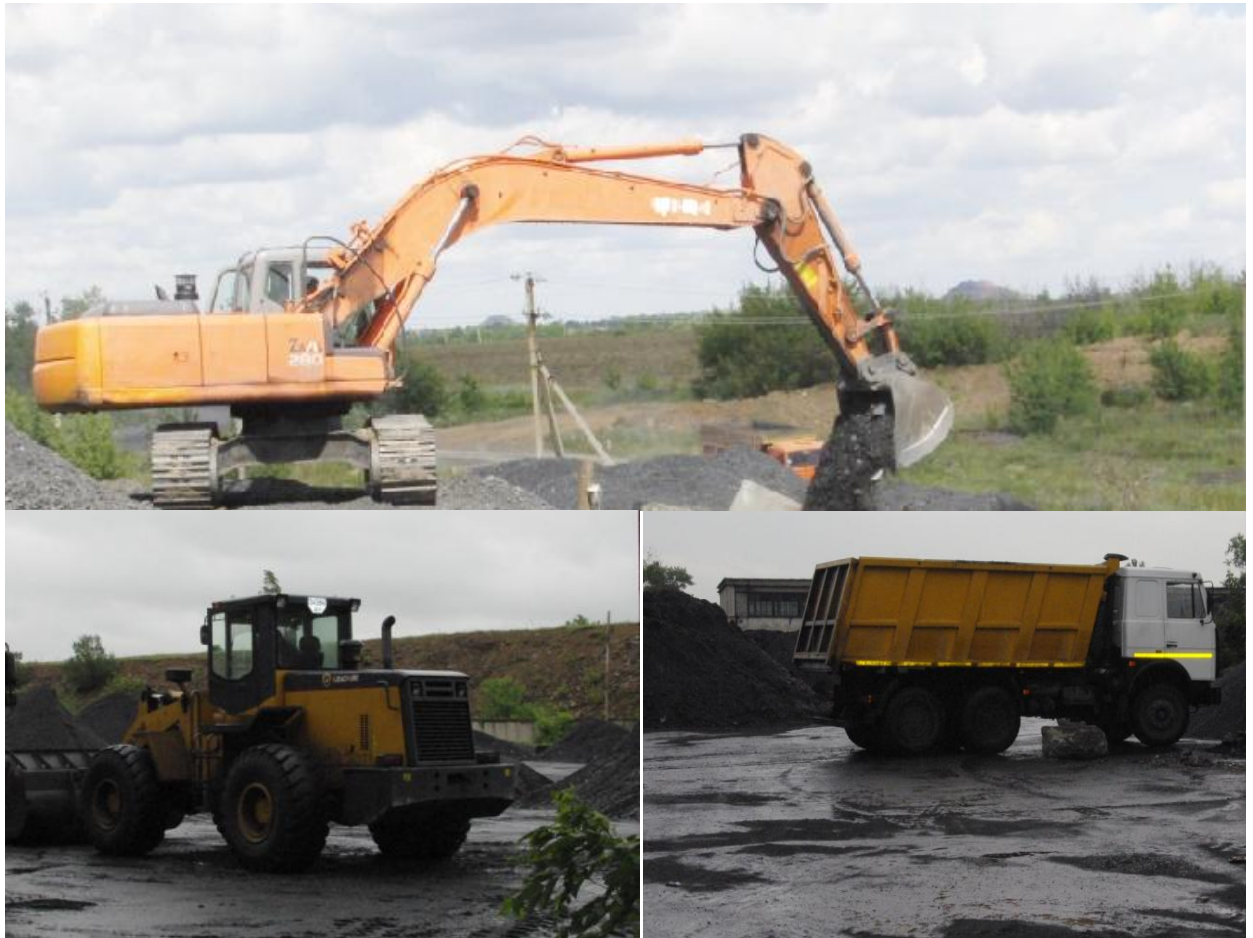
Figure 5 - Machinery involved in the project.
