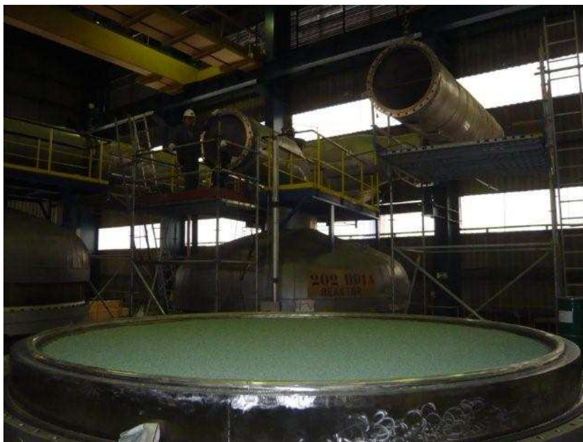
Figure 2: Installation of secondary catalyst
