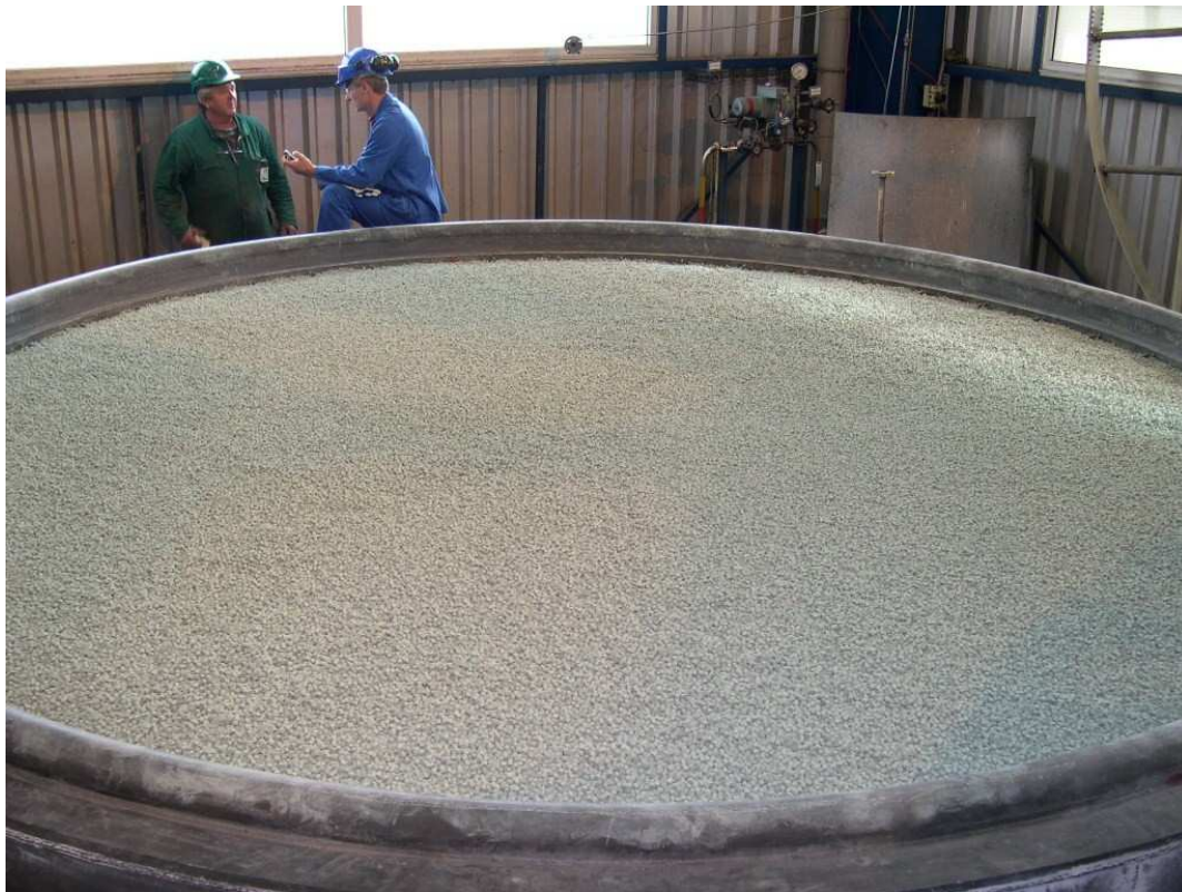
Figure 2: Installation of secondary catalyst
