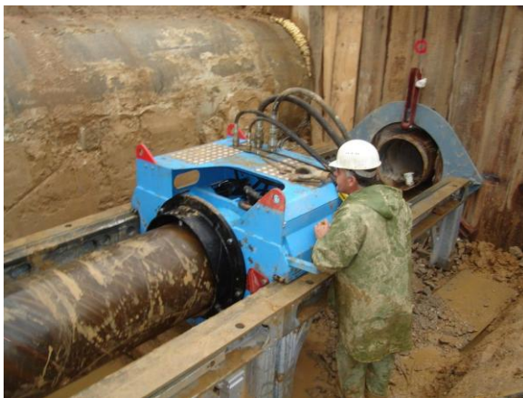
Figure 4. Operation of horizontal drilling machine
