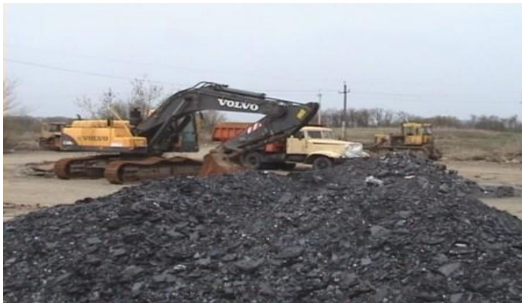
Figure 5 – Special technique that dismantles waste heaps and transports rock mass
