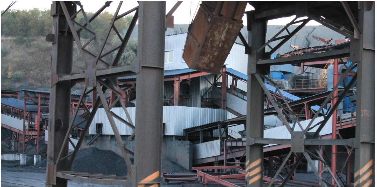
Figure 6 – General view of the complex for processing the rock mass of the waste heap
