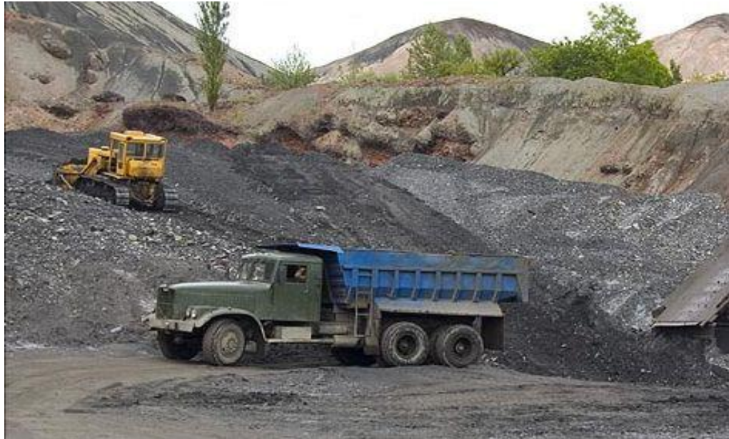
Figure 4 – Demonstration of conducting works on waste heap dismantling
