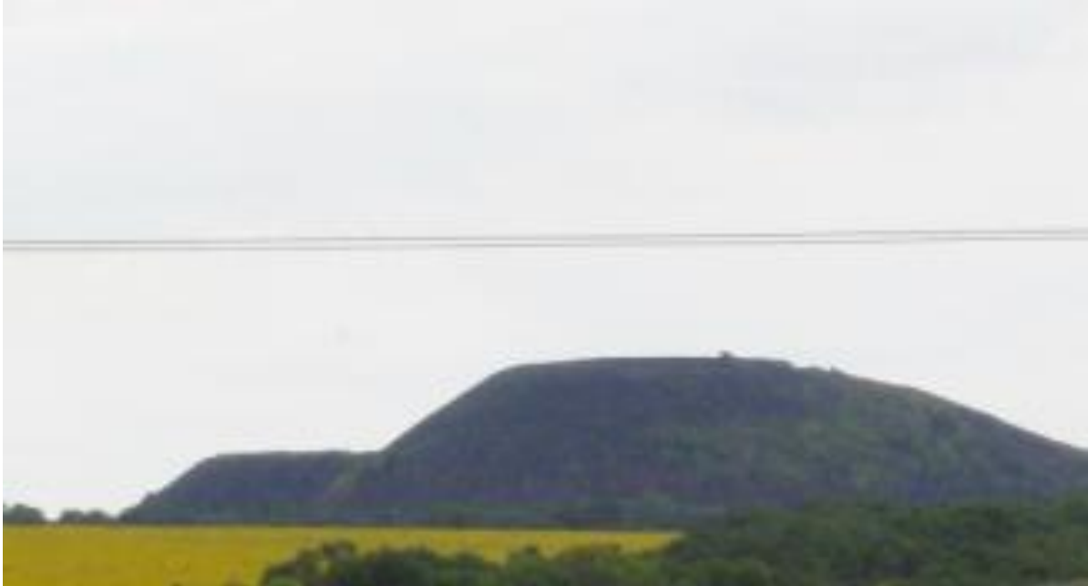
Figure 2 - The exterior of the waste heap under stage of dismantling
