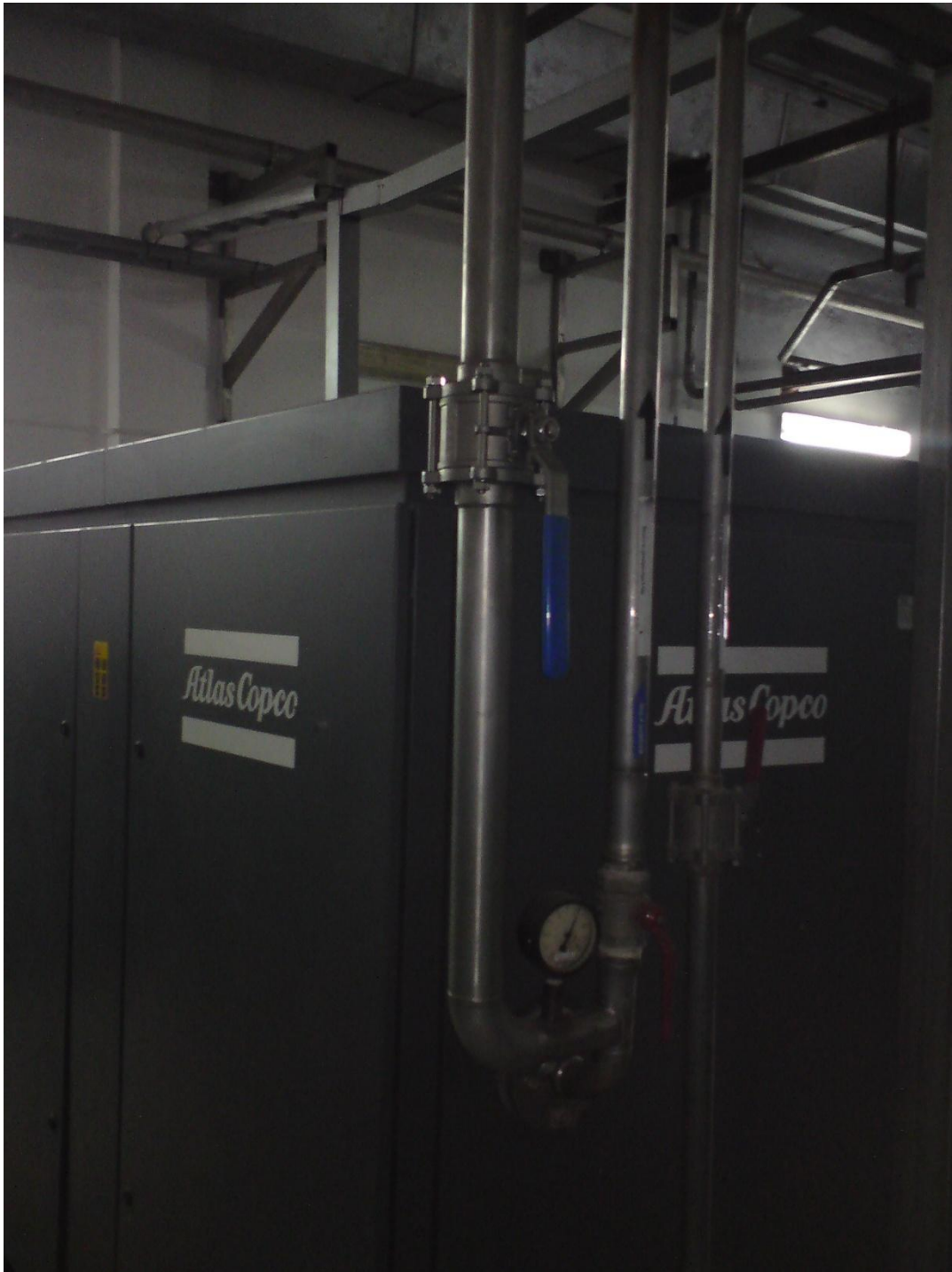
Figure 14 – System of compressed air pipelines
