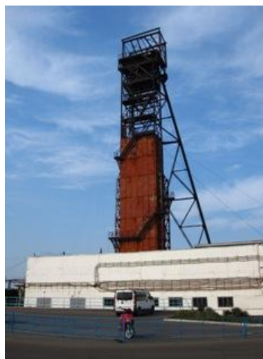
Fig.3 A shaft of Coal Mine named after M.P. Barakov.
