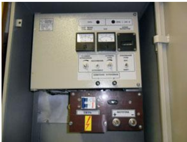
Figure 6. Appearance of a cathodic protection plant “Elkon” and basic scheme of cathodic protection: 1 – gas pipeline, 2 - anode electrode, 3 - cathodic protection station
