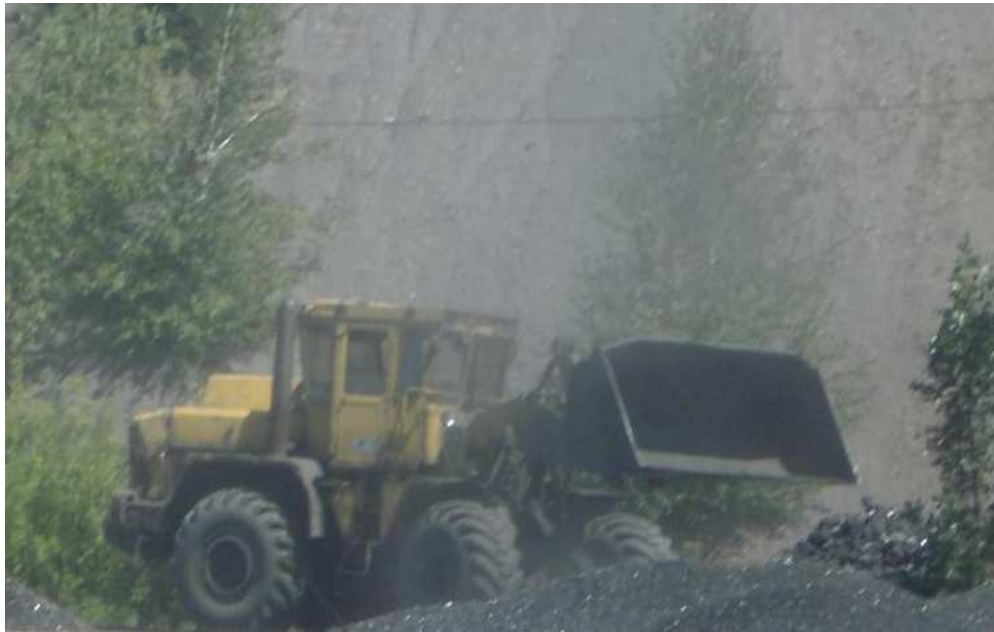
Figure 4 – Technology that dismantles a waste heap
