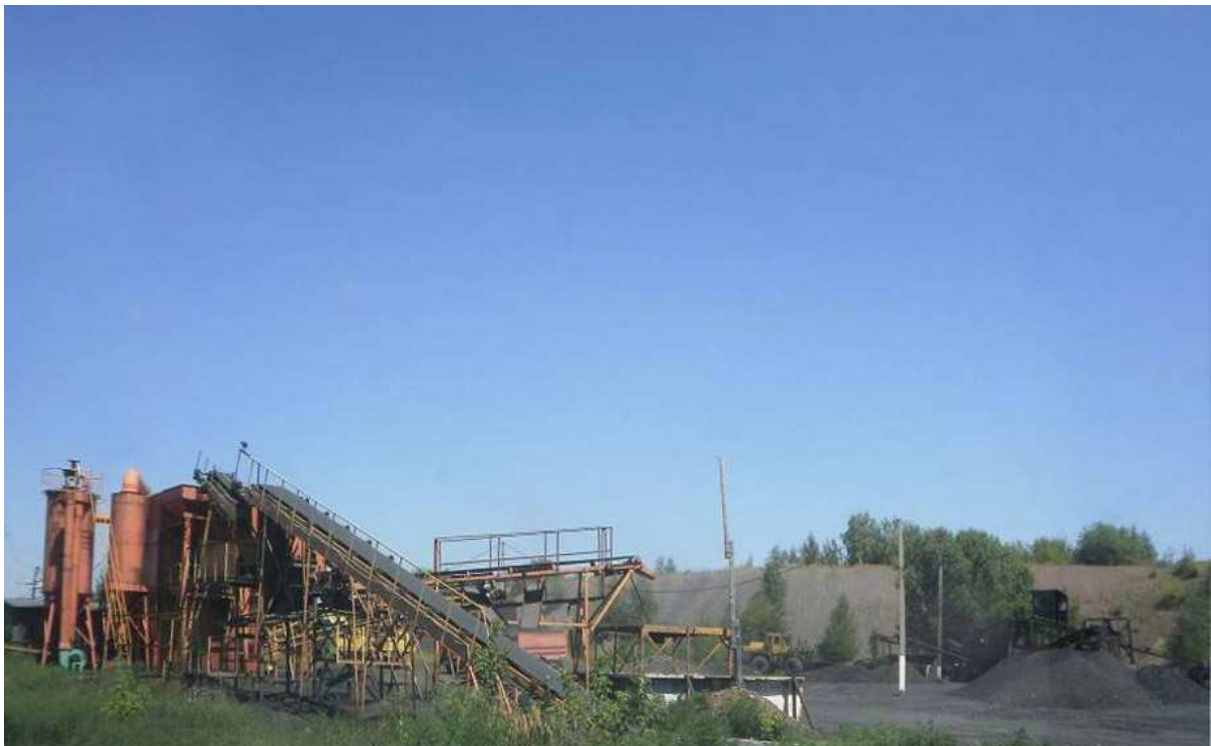
Figure 5 – General view of the complex for processing rock mass of the waste heap
