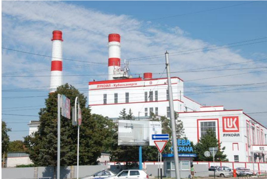
Fig. A.3-1. Krasnodar CHPP of LLC "LUKOIL-Kubanenergo"
