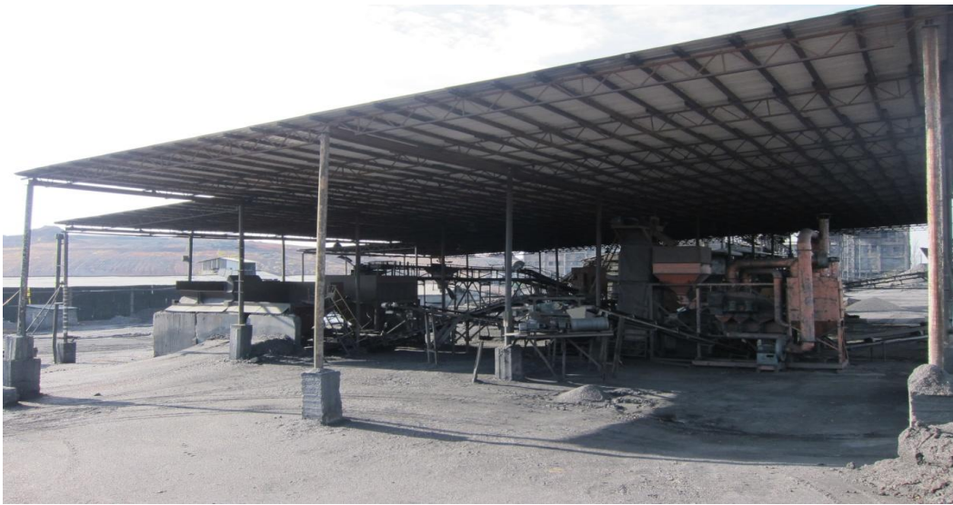
Figure 3 - CEP “Tsentralna” involved in the project
