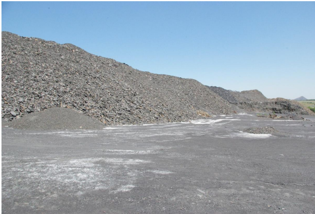
Figure 2 - The exterior of waste heap under dismantling stage
