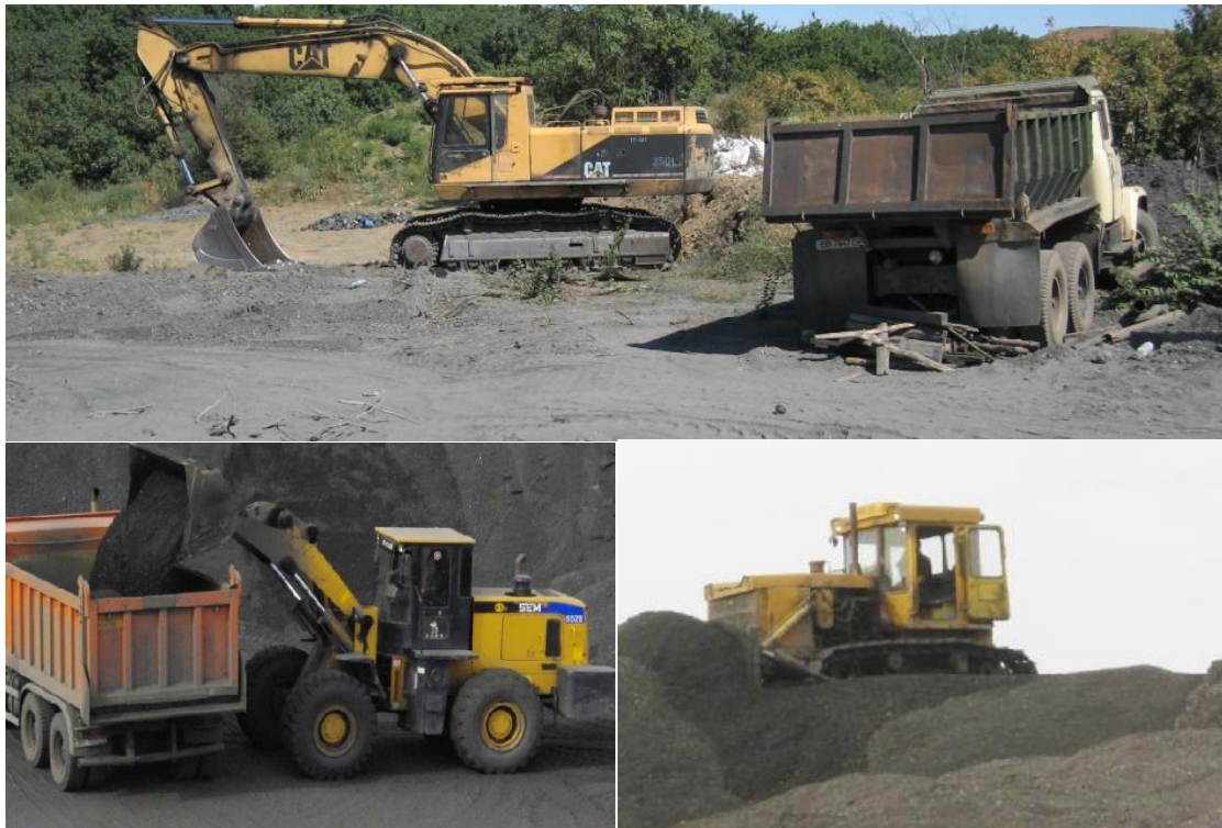
Figure 4 - Machinery involved in the project.
