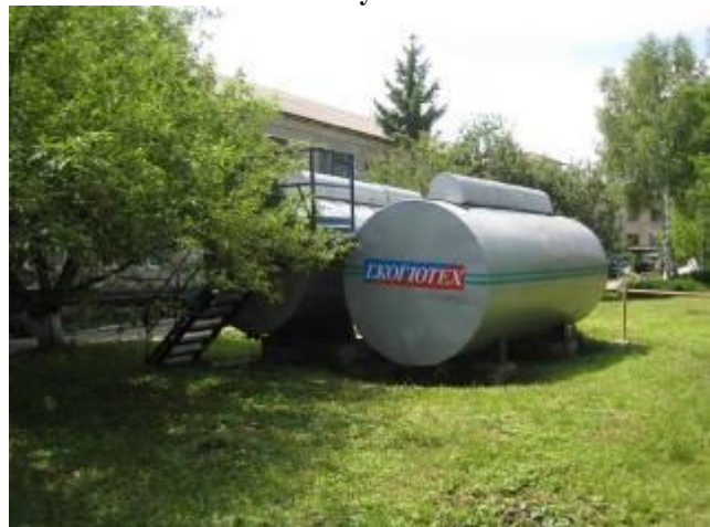
Electrical heating of the hospital and the sanatorium with the heat accumulation at night and its usage during the day. Stara Ushytsya.
