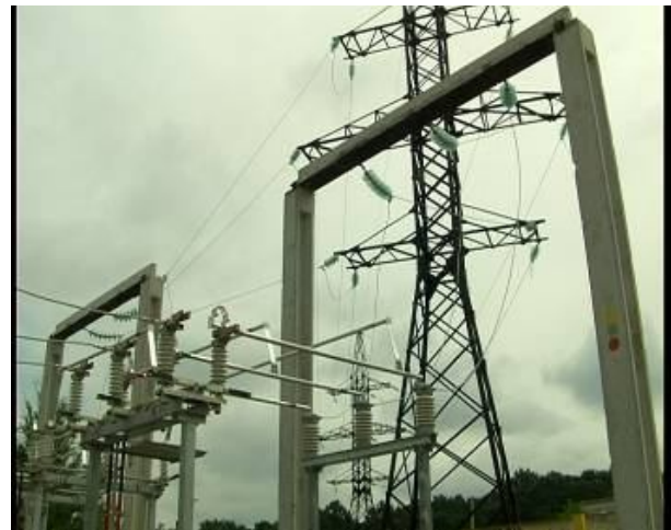
SS-110/10 kV «Krystal». Gantry and line discharger after the installation.
