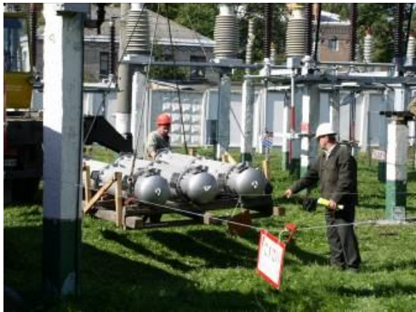
SS-110/10 «Tsentralna». VRU-110 kV. Installation of a gas-insulated switch (Siemens production).
