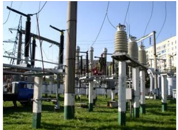
SS-110/10 kV «Krystal». VRU-110 kV after the construction.
