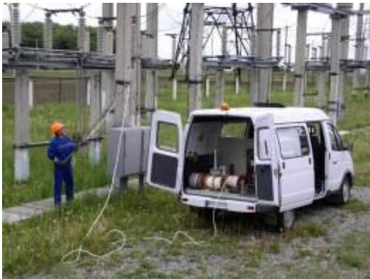
SS 110/35/10kV «Yarmolentsi». Transportable control laboratory TCL-110. Current transformers control 110kV without their dismantling.
