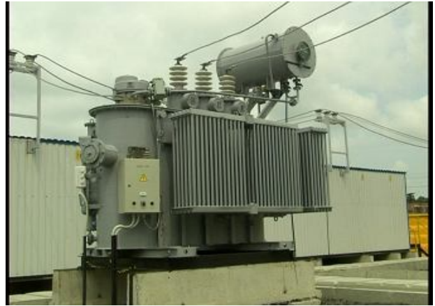
SS-35/10 kV «Elevator». Power transformer (2,5 MVA) after the mending.
