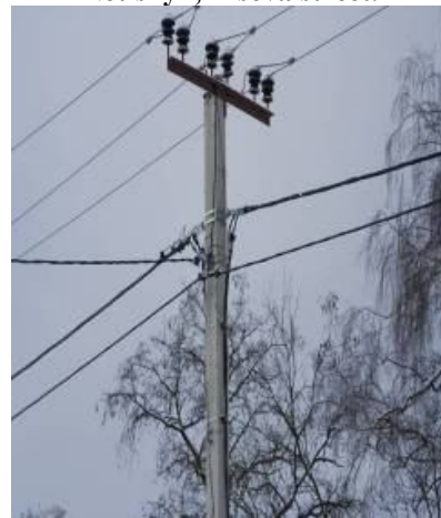
Inlet with isolated wire in the dwelling house. Netishyn, Lisova street.
