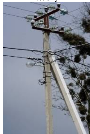
Electrical networks reconstruction for electrical heating. Netishyn.
