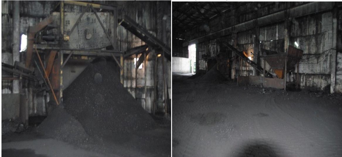
Figure 4 - Machinery for sorting rock mass
